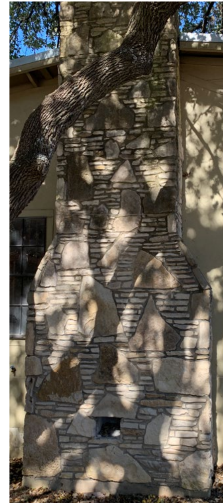
Existing masonry chimney
