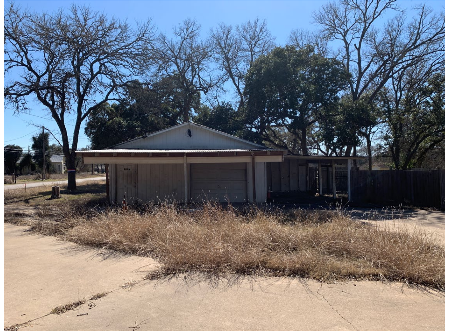
Existing garage to be removed.
