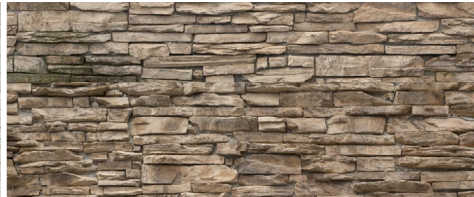
Flagstone at base
