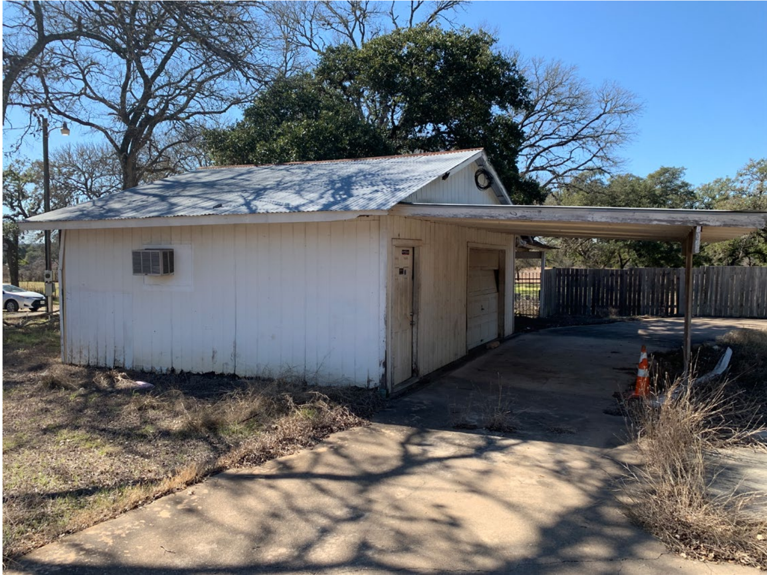
Existing garage to be removed.
