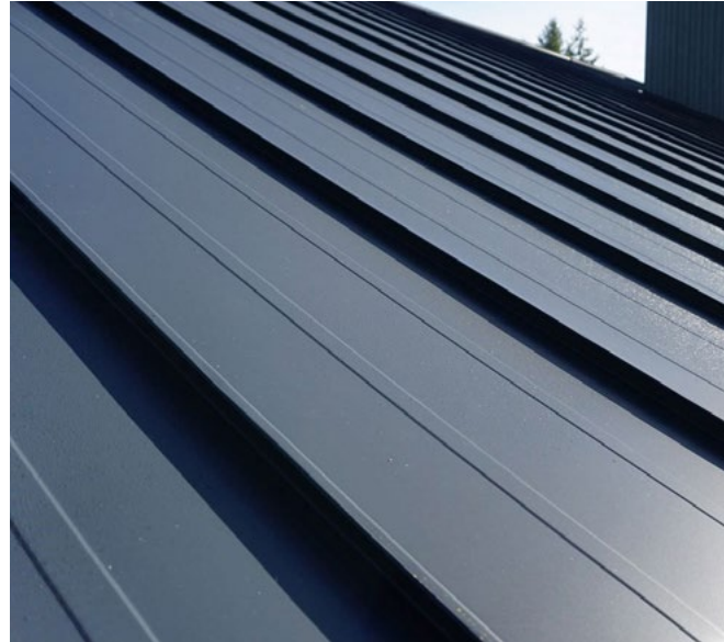
Standing seam metal roof.
