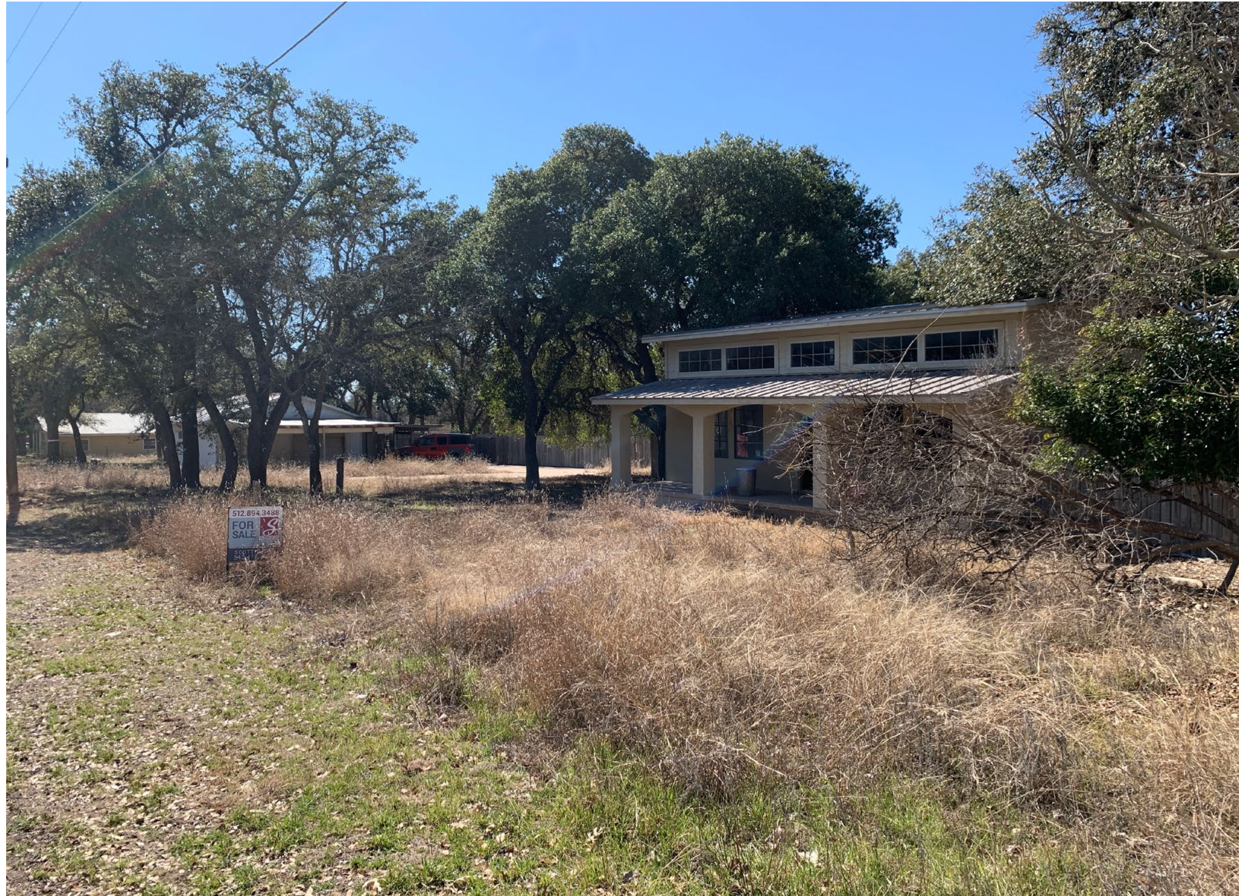
Existing homestead from Old Fitzhugh Road
